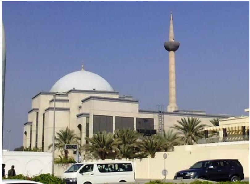
Client's strict requirements of “no noise disturbance for neighbors” and “no equipment to be located on roof” required an innovative design using split units with centrifugal condenser fans located in the basement. Condenser air discharge through grilles integrated into the façade architecture (in picture above). The unique interior design required supply via jet diffusers.
